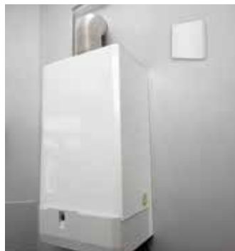
Bathrooms & rooms with boilers
