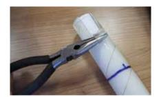
Using long nose pliers, grip the end and roll the PU back to the mark. Repeat this until all the outer is peeled back.
