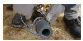
Stainlees steel hose clamps are used to clamp the inner pipe of ProtectaFlex Detect to realize the jointing with plastic fittings or, eventually, to clamp the outer pipe of the solution.
