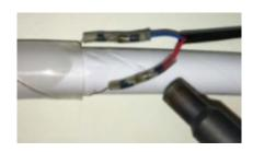
Heat the sleeves until they have shrunk completely and the solder rings have melted and flowed. Keep the heat source moving to avoid charring. Do not move the joint until it has cooled, this may weaken the joint.
