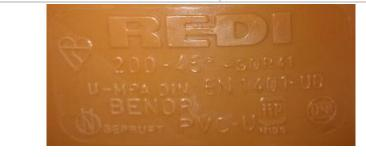
\* UD: application area code for non-pressure underground drainage and sewerage for both buried in ground within the building structure and outside the building structure
